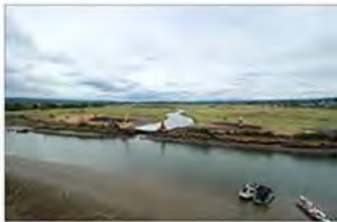
Crew opening Ebey Slough levee, Qwuloolt Estuary, August 28, 2015, 12:15 p.m.
