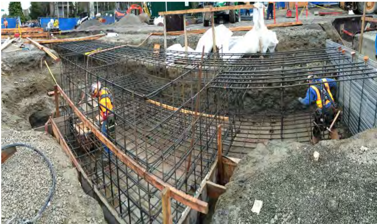
Rebar cage for the mat footing and elevator pit.
