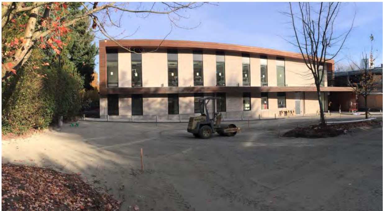
. . . to near completion.
