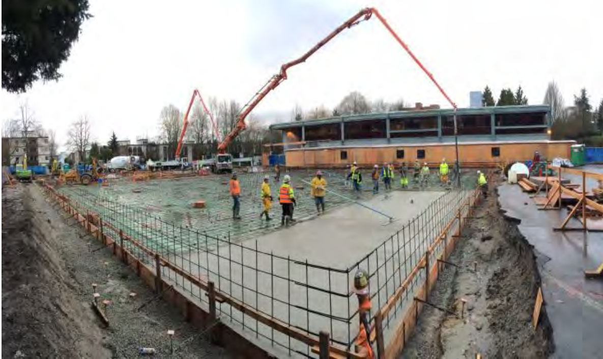
Slab on grade placement day.
