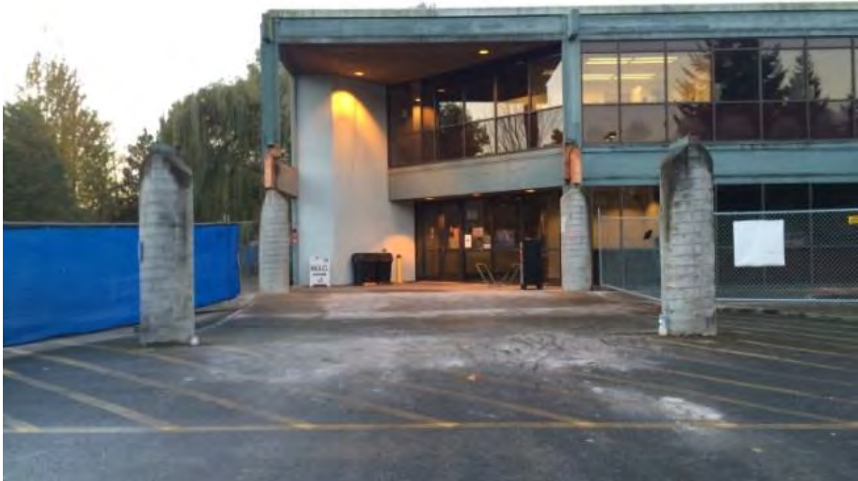
Main Entrance to the North Public Health clinic after canopy removal.
