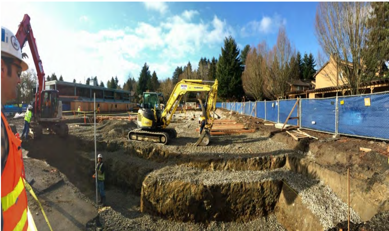
Looking Westward across the site at the structural excavation for the foundation work.
