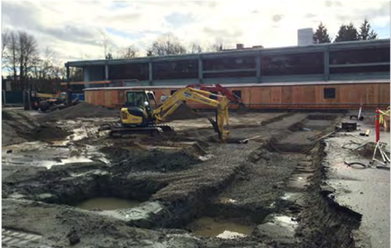
Looking Southeast across the site during structural excavation.
