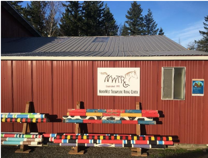
New Barn Roof
