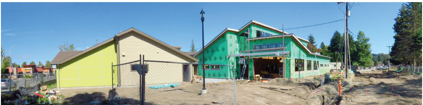
Current construction progress for the Phoenix Rising project, September 15, 2015.
